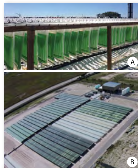
▲ Figure 7.6: Photobioreactor farm established at Algenol, Ft. Myers, FL, USA, (A) hanging bags designed to collect the headspace, (B) large-scale integrated algae-ethanol-producing farm
